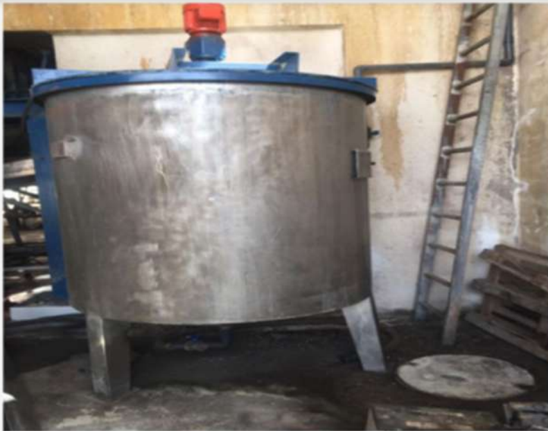
Figure 12: Additional pretreatment unit
