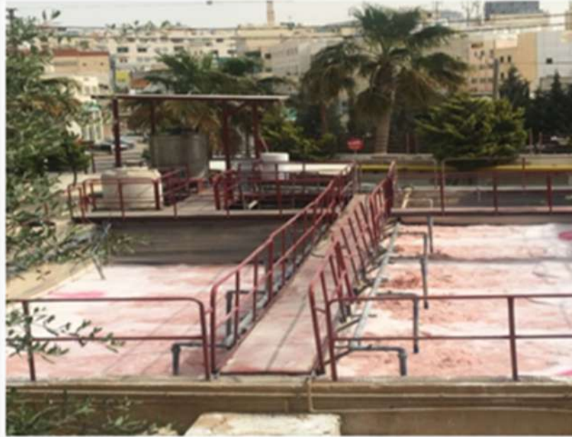
Figure 15: pretreatment units for pharmaceutical factory in Jordan
