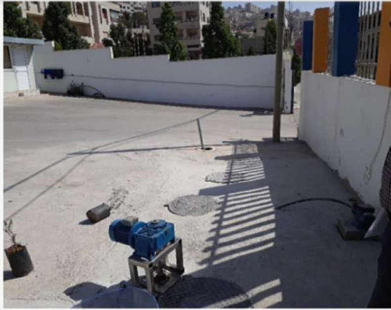
Figure 11: Pre-Treatment Unit at Dana Veterinary Factory
